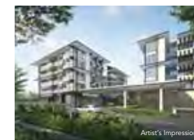
SINGAPORE THE VERANDAH RESIDENCES
