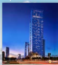
CROWN STREET ELIZABETH TOWER Completing Q1 2022
